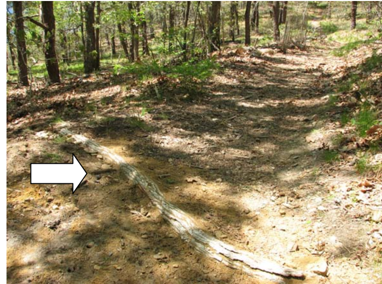
Right- Water bar installation
